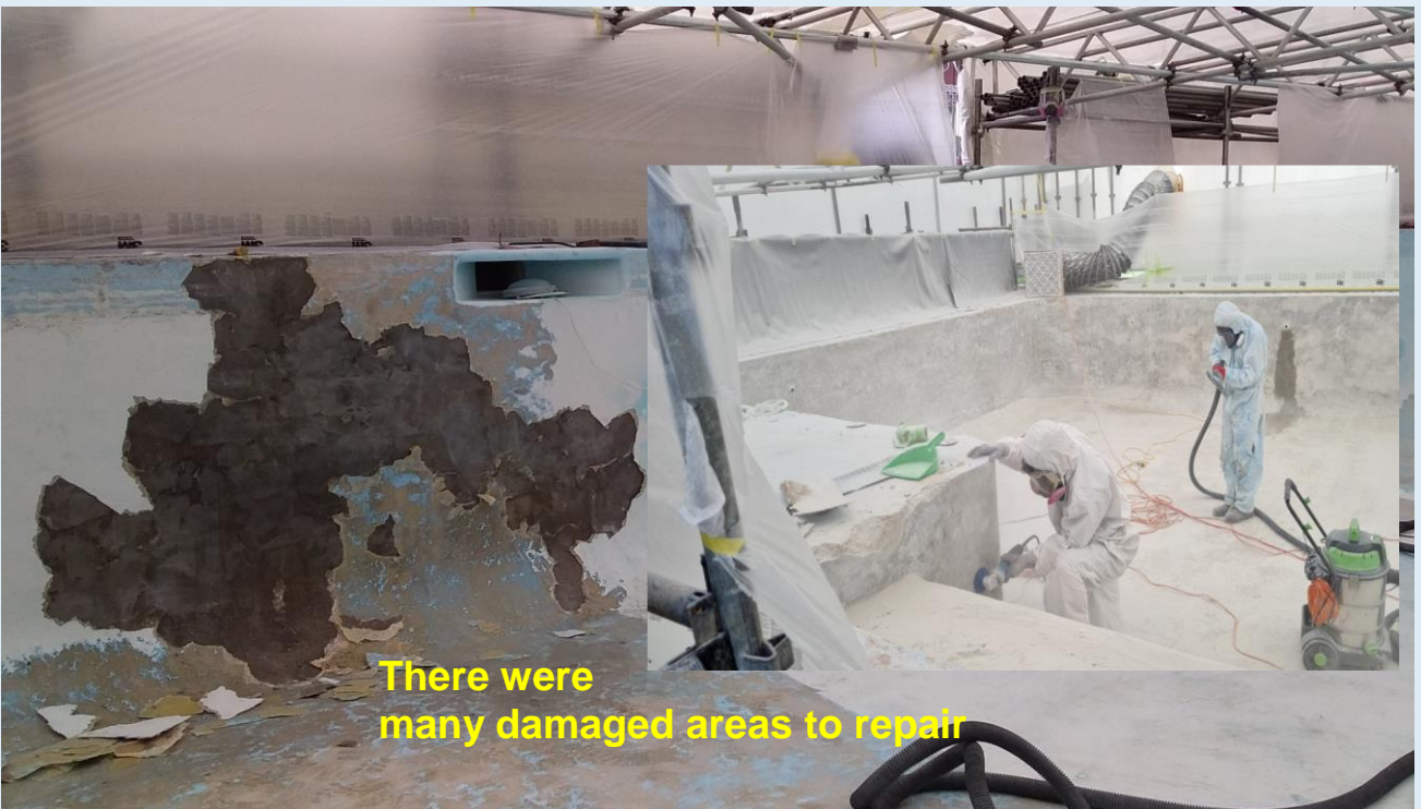
The technical work underway inside the created workroom
